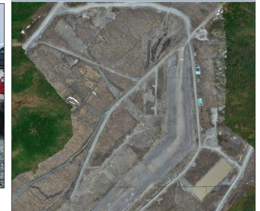
TMF Dam Overview
