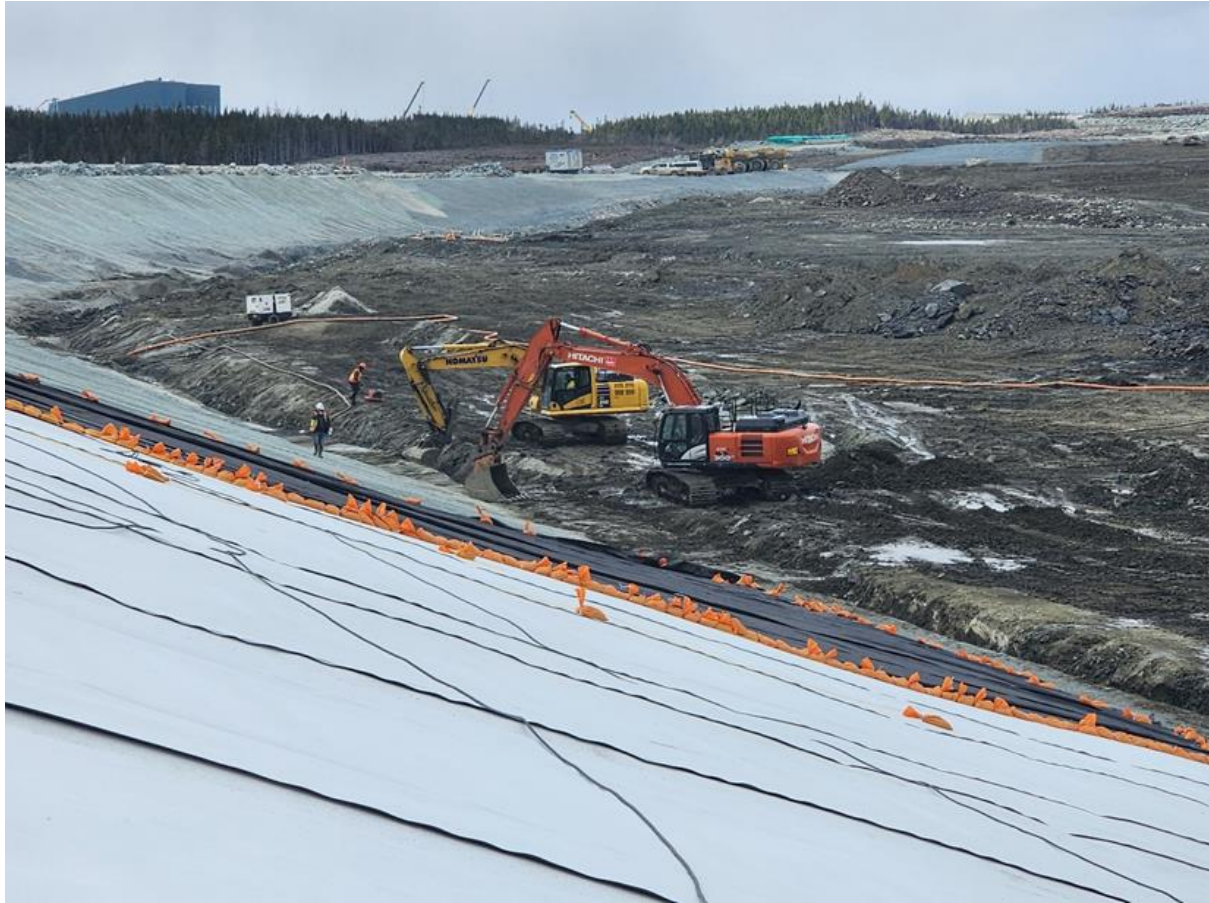
Tailing Management Facility Anchor Trench Construction
