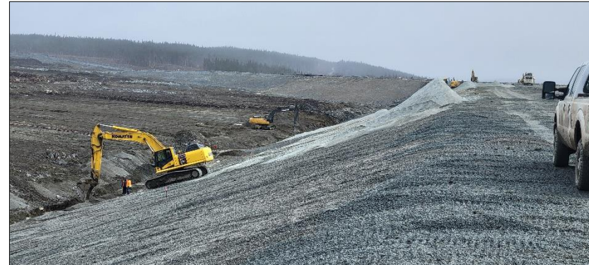
TMF Dam Construction
