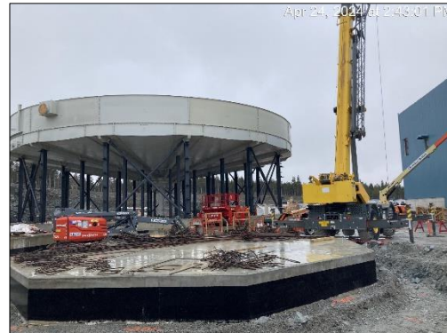
Thickener structural steel / infill segments installation
