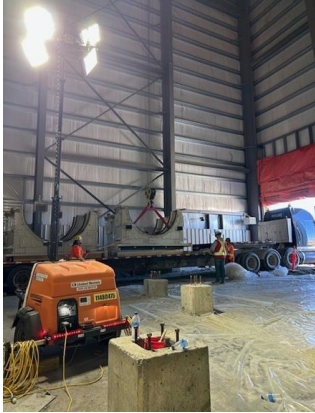
Off-loading trunnion bearing bases using the OH crane
