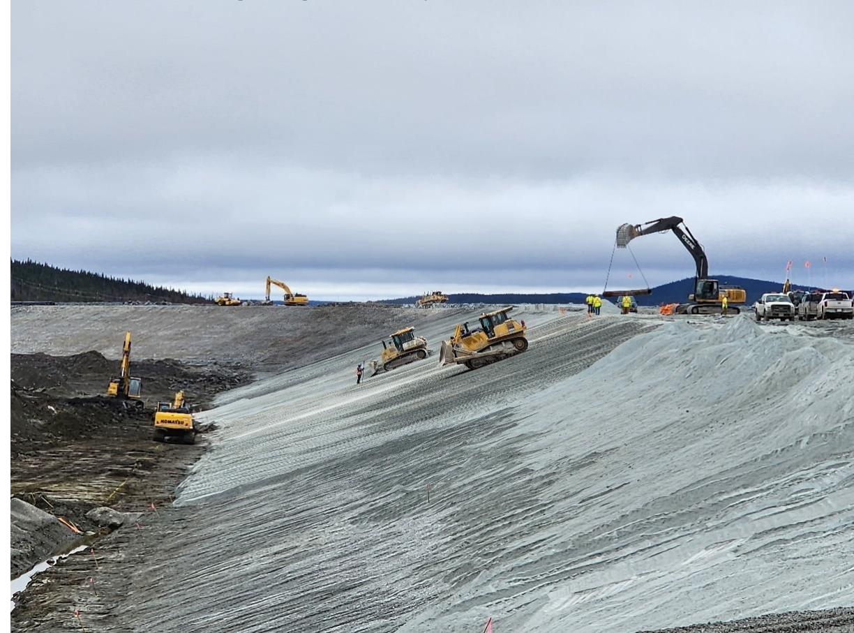
Tailing Management Facility Embankment Construction
