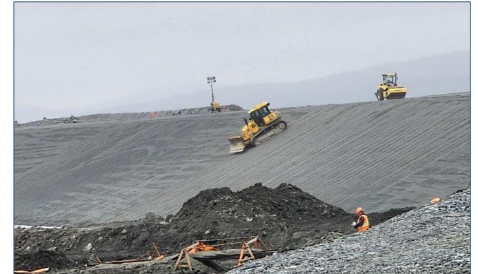
TMF Dam Construction
