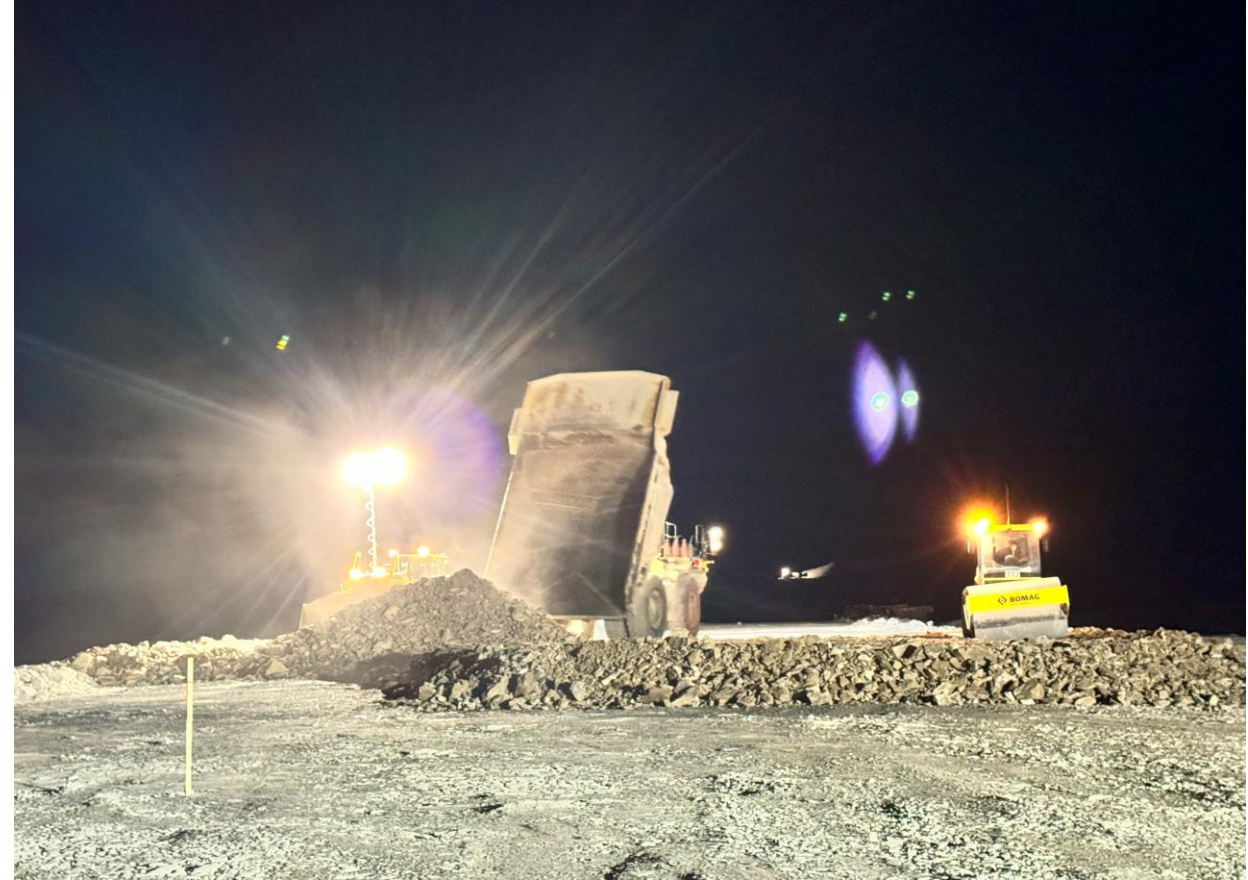
Tailing Management Facility Rock Placement
