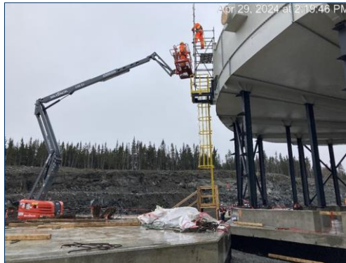
Thickener structural steel / infill segments installation
