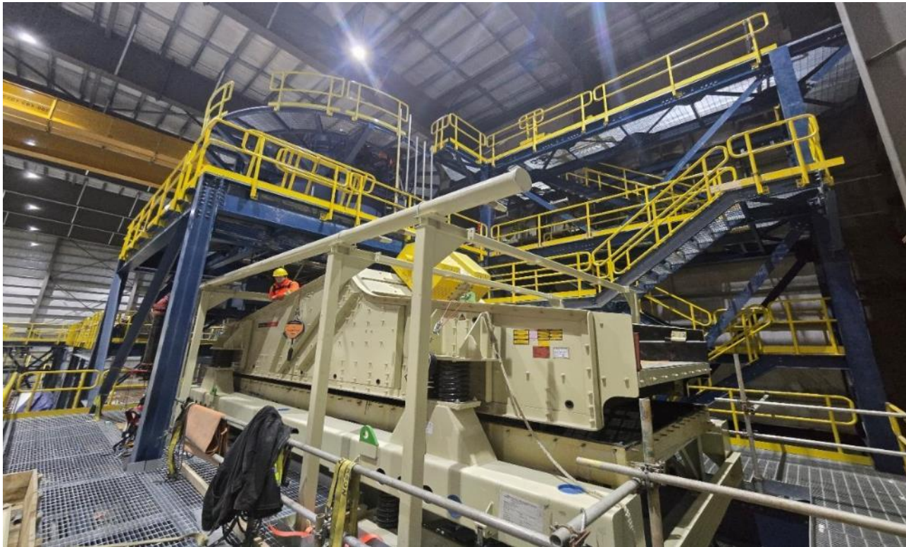
Mechanical Installation - Oct 2024
