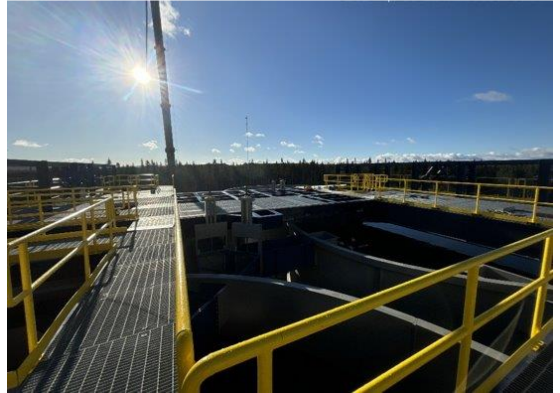
Bridge Installation - Oct 2024
