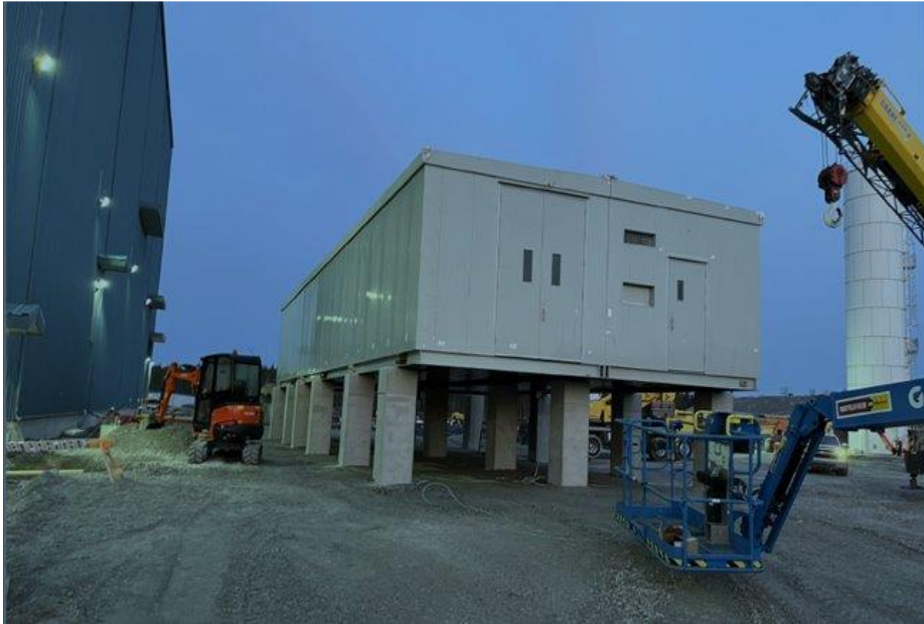
General E House Set in Place – Sept 2024
