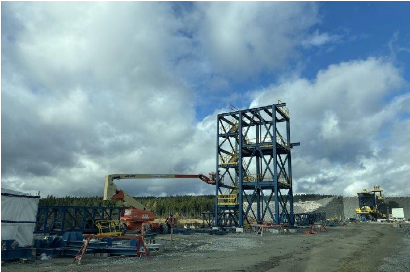
Conveyor Construction – Sept. 2024
