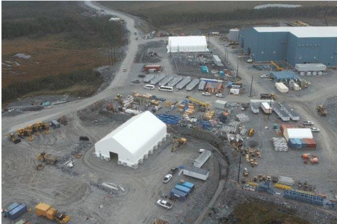
Warehouse Building and Plant Site – Oct. 2024
