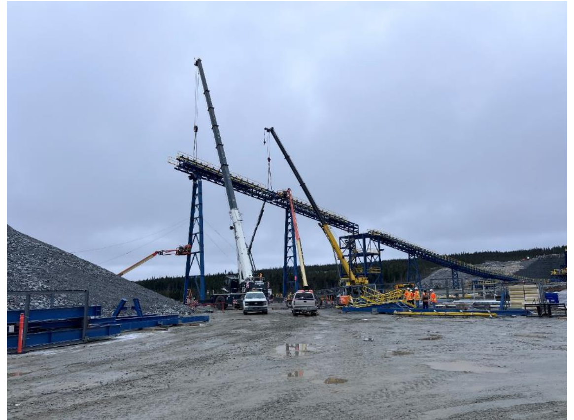
Conveyor Construction – Oct. 2024
