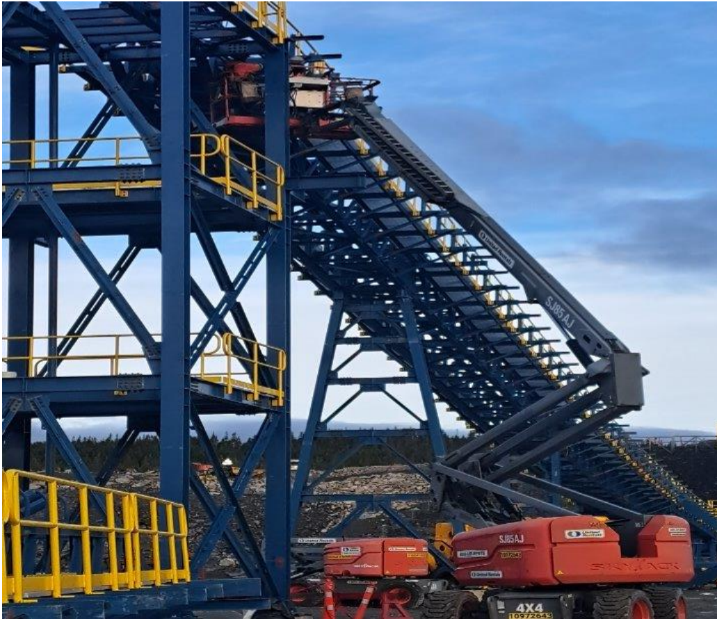
Conveyor Construction – Oct. 2024
