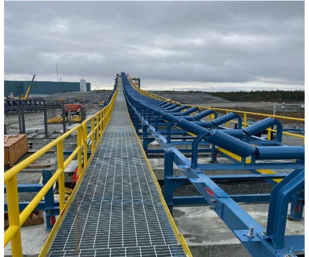
Conveyor Construction – Oct. 2024
