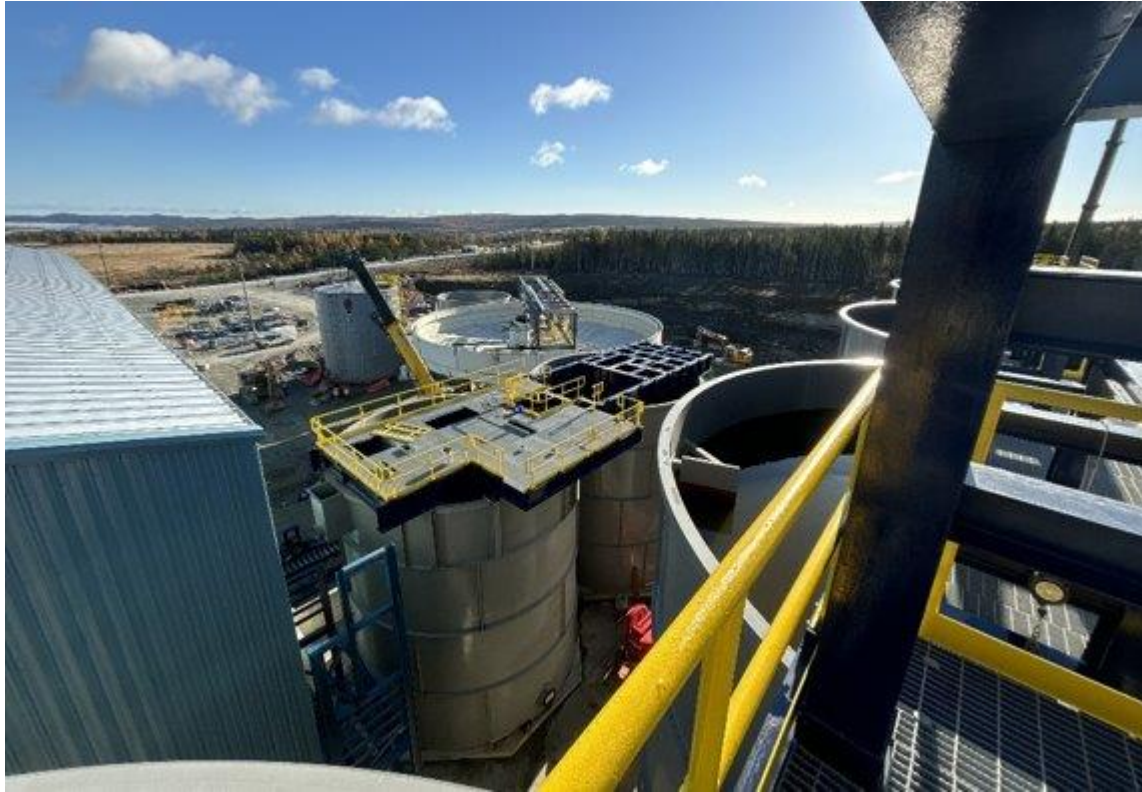
Cyanide Detox Bridge Installation - Oct 2024
