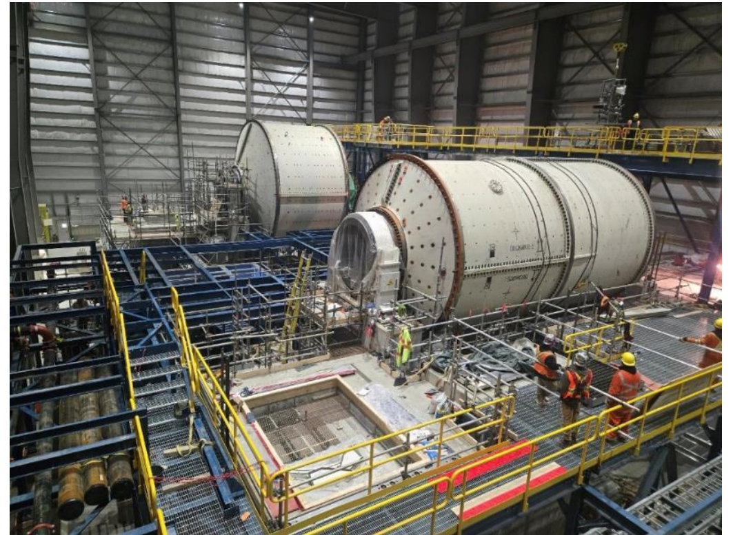
Ball Mill Motor Foundation - Oct 2024
