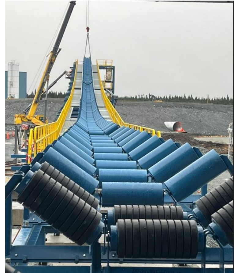
Conveyor Construction – Oct. 2024
