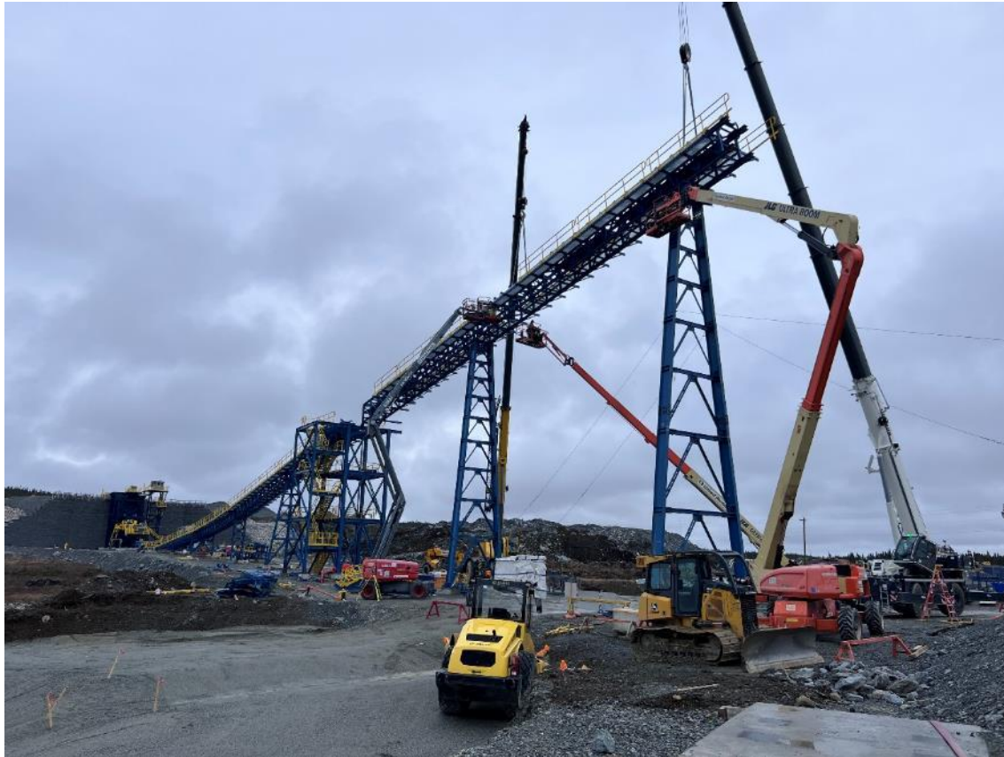
Conveyor Construction – Oct. 2024
