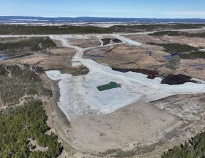
Civils work underway at the future process plant site. On the left, a NW view showing bedrock blasting on the left and the haul road and Leprechaun Mining pit in the far background. On the right, a NE view showing the haul road and overburden stockpile location in the background. Both photos April 2023.
