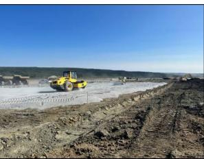
Figure 4: Construction of the TMF. Spreading Filter Layers for Geomembrane Liner Placement. September 2023
